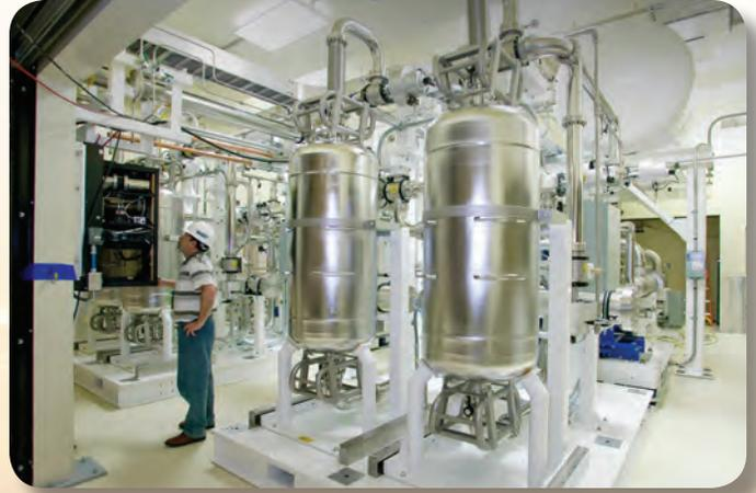
A state-of-the-art tritium-processing system has been installed to contain very small amounts of tritium in NIF targets and provide a mechanism for its safe disposal. More than \$300,000 per year is saved through optimized tritium processing operations with infrequent exchanges and recycling of the tritium collection vessels.
